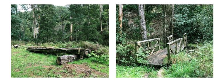
Billy's Weir can only now be accessed if walkers enter the creek. Over the years with many storm events the Weir is silting up. The area behind the weir is getting shallower and is now only a few feet deep. In the center of the weir the silt has collected and now makes a solid bank above water level.
