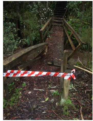
The bridge across to Stringybark track has been cleared of many fallen trees, but sadly the bridge has been damaged and will need massive repairs or replacement. (The first photo is from June 2021 and the other photos are from this month.)
