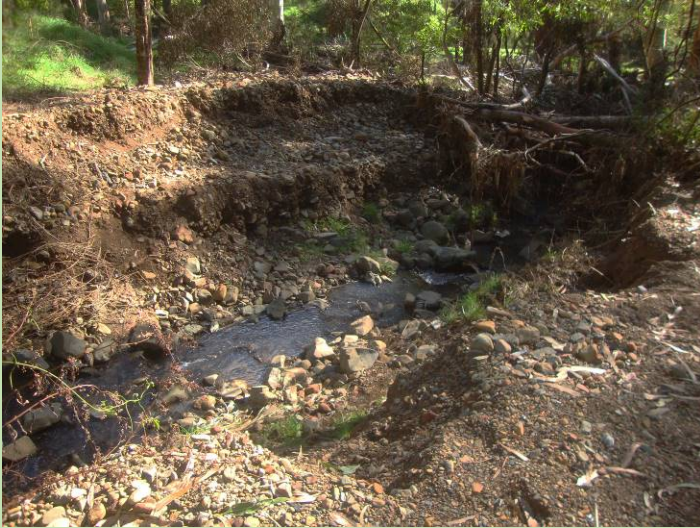
The first creek crossing to Blue Gum Hill. It is now a deep ravine requiring a lot of earth and rock movement or a bridge if walkers are to cross safely.
