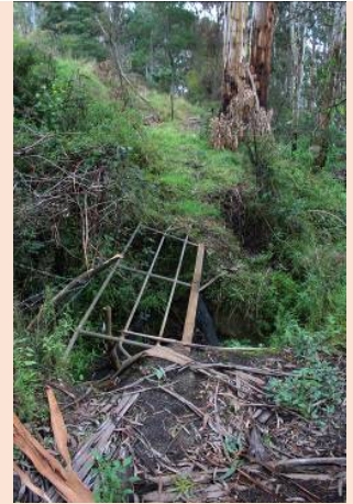
The crossing over the dam overflow has burnt away and the hand rail is now across the gap. If this track is to be used a new crossing will need to be made.
