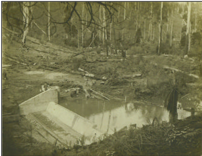
Weir under construction Photo: by ? Date: c. 1913
