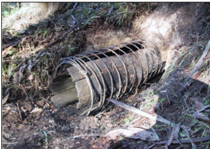
Remains of old pipe-line Photo: by Hilmar Batza Date: 20-07-03
